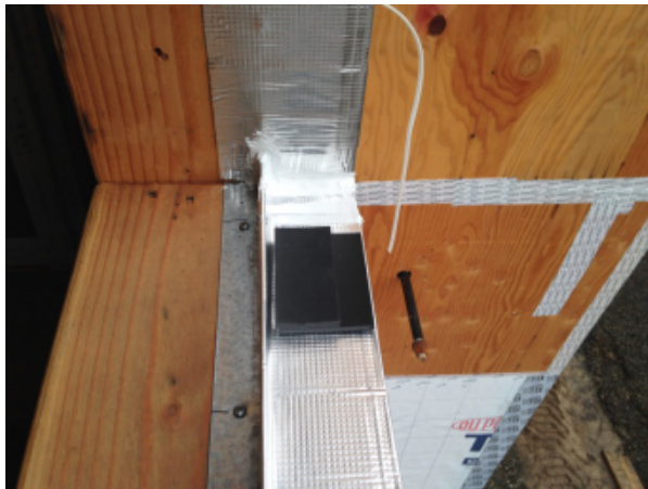
Fig. 34 - View of sill pan showing two-stage shim. This set-up allows the metal sill flashing to enter the gap between the sill pan and the window frame.
