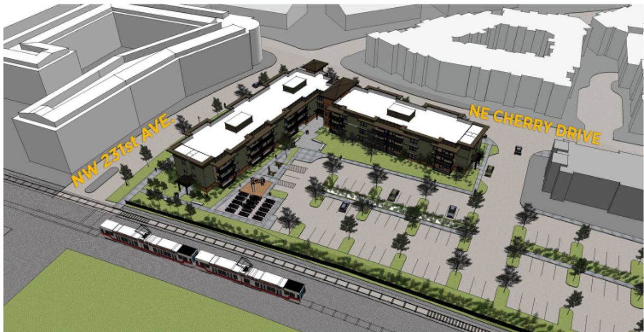
Fig. 2 - Aerial view of the site and building. Note the three penthouses at the roof which house the mechanical equipment and are included within the Passive House enclosure. Image courtesy of Ankrom Moisan Architects
