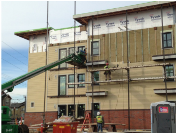
Fig. 50 - Fiber cement siding and trim installation in progress.
