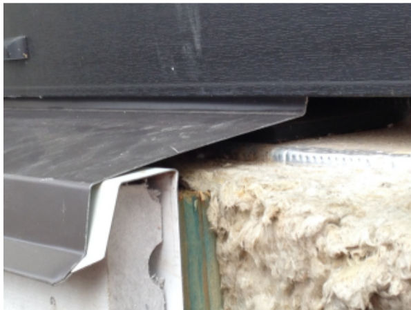
Fig. 46 - Metal sill flashing (at mockup). The flashing is inserted into cavity at underside of window frame. Bond breaker tape and sealant is then applied at the gap. The flashing is placed on the lower of the two shims to provide support and maintain free drainage from the sill pan area.
