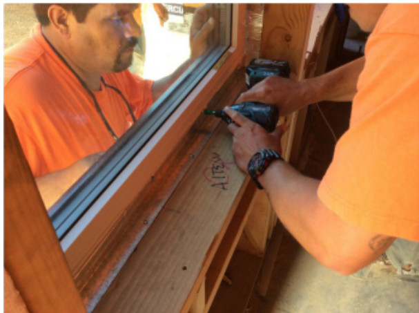
Fig. 36 - Window is fastened at the sill using an aluminum angle provided by the window manufacturer. The angle also serves as support for the SAM sill pan.
