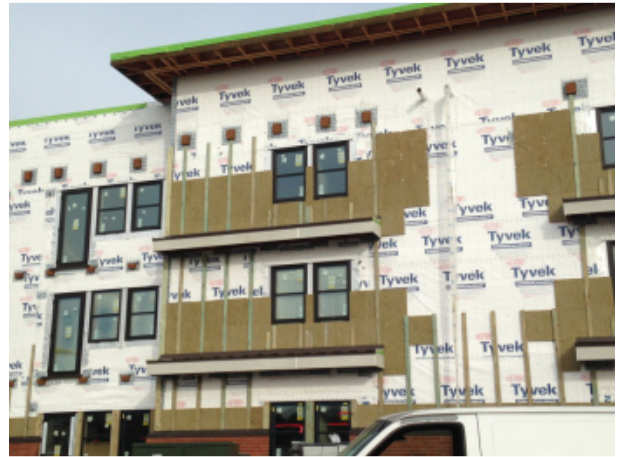
Fig. 49 - Mineral wool exterior insulation and treated wood furring installation in progress.
