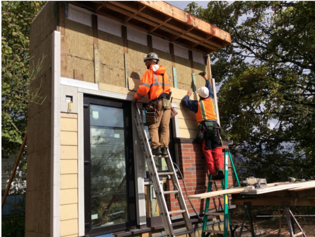
Fig. 8 - Exterior wall mockup
