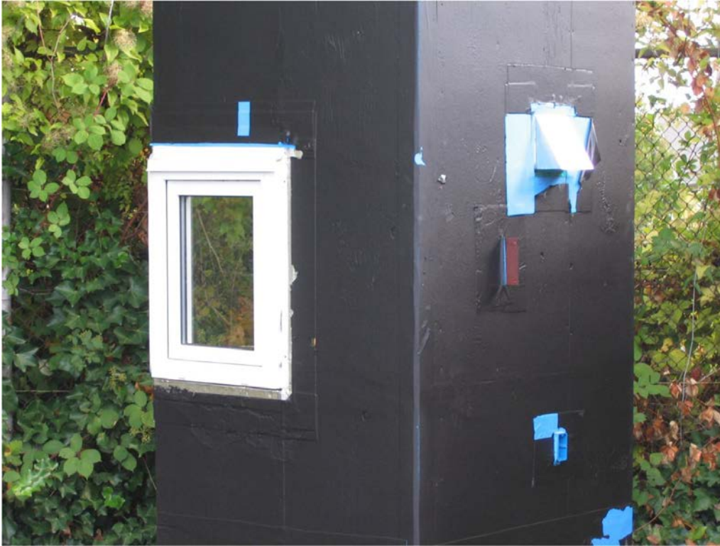
Figure 2. View of mockup after adhesion testing conducted 10 days after demonstration.
