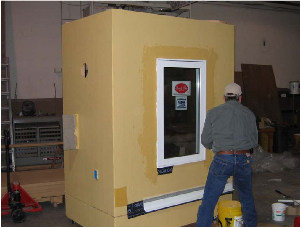
Figure 3. Installation demonstration by alternate liquid-applied membrane manufacturer.
