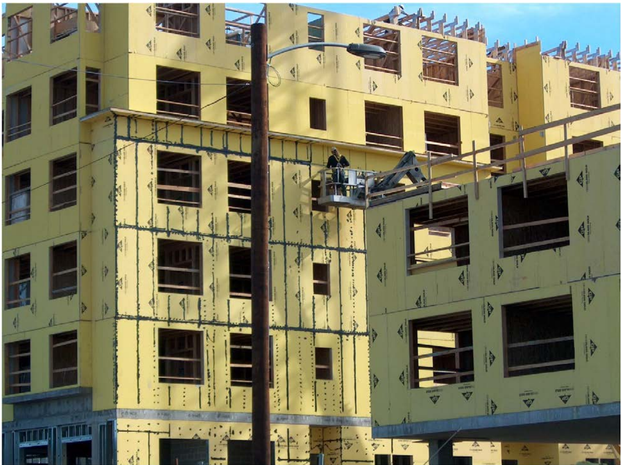
Figure 5. Exterior side air barrier during installation.
