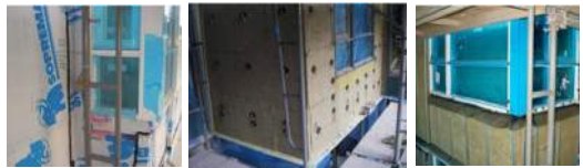
Post-Rehabilitation - Exterior Membrane & Fully Exterior Insulated
