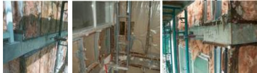
Post-Rehabilitation - Exterior Membrane & Fully Exterior Insulated
