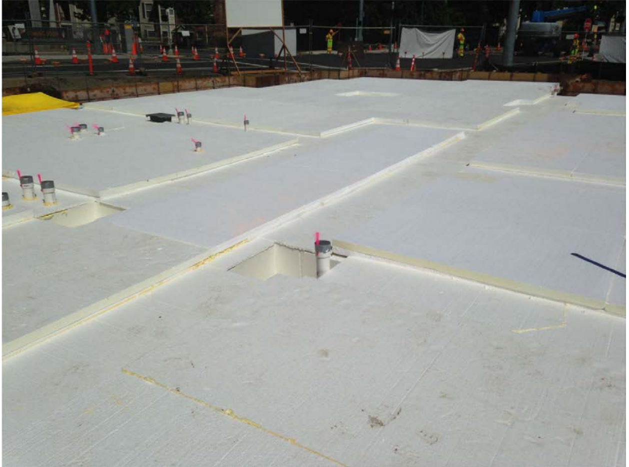
Slab insulation installation in progress.
