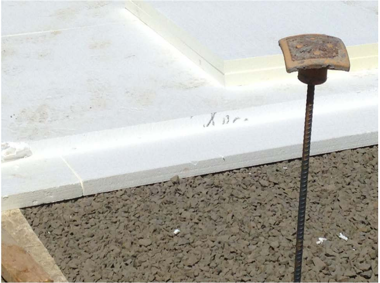
View of foam insulation layers installed over the compacted gravel base.
