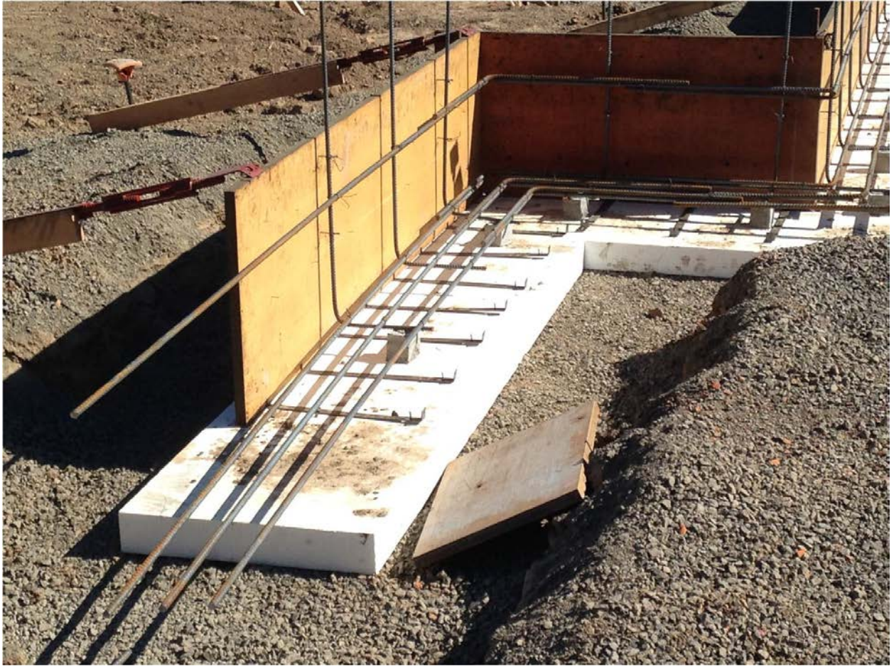
Footing formwork in progress.
