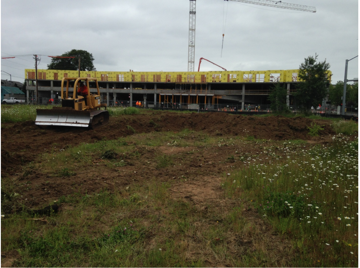
Breaking ground, moving dirt!
