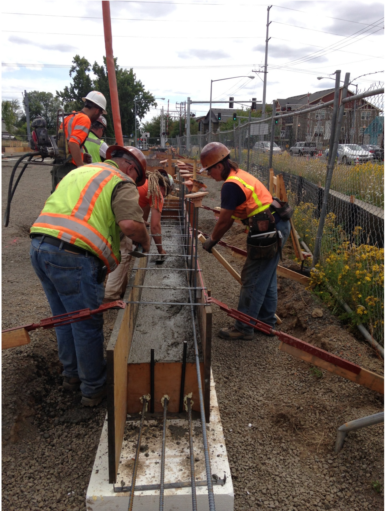
Troy and team finish the mud as it is placed. Denise braces the forms.
